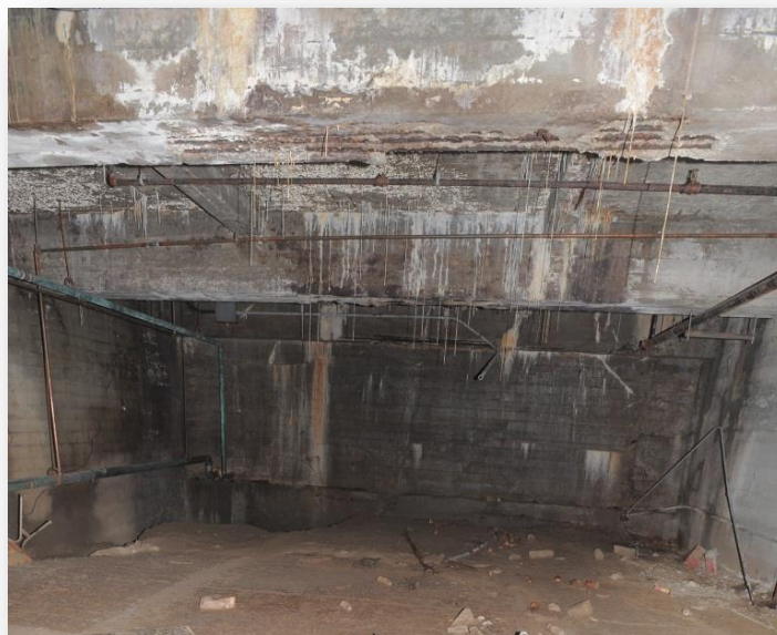
Water damage to substructure and foundation (Source: Tim Bommel)
