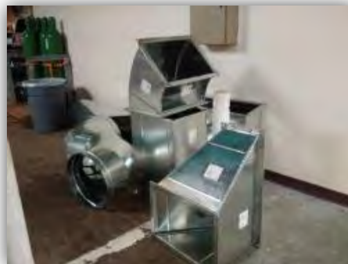
Replacement ductwork awaiting installation; one component of the first phase of the HVAC upgrade.
