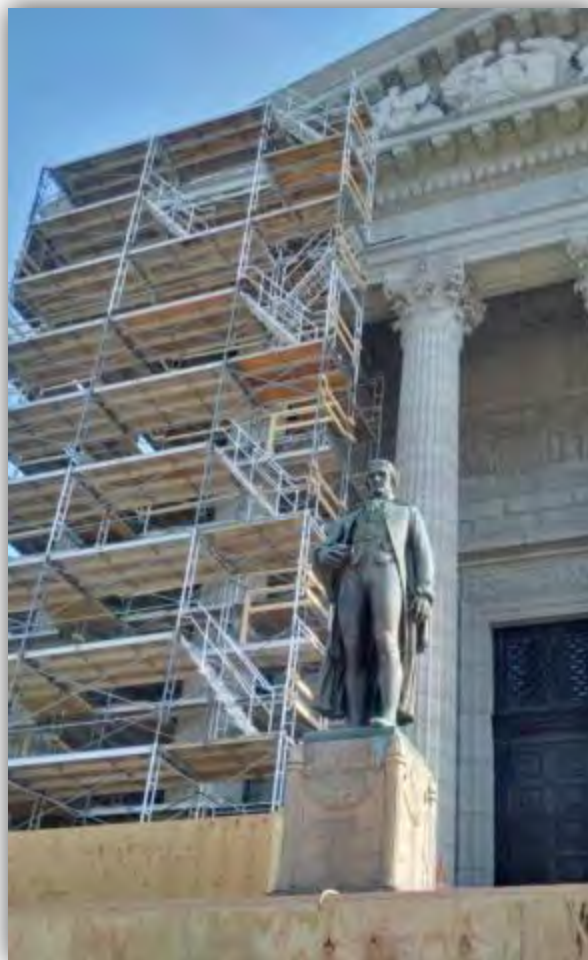
Scaffolding arises at the south entrance in preparation of assessment of the stone pediment - September 2015
