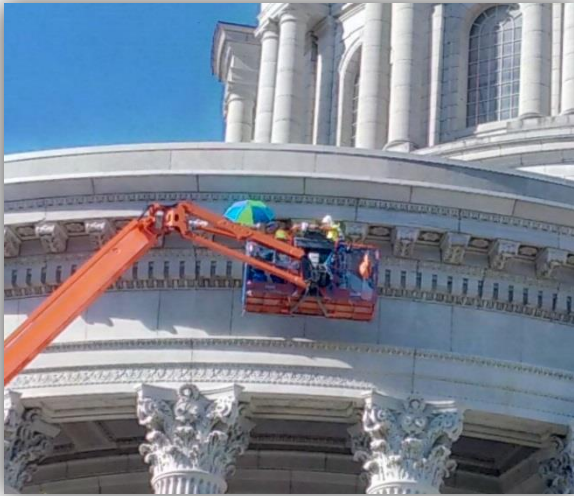
Workers examine and make repairs to the stone dentil molding on the Capitol's north portico
