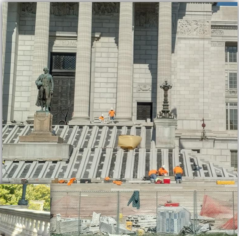
Continued progress on the south stairs and plaza areas as workers install the new waterproofing membrane. (above)
