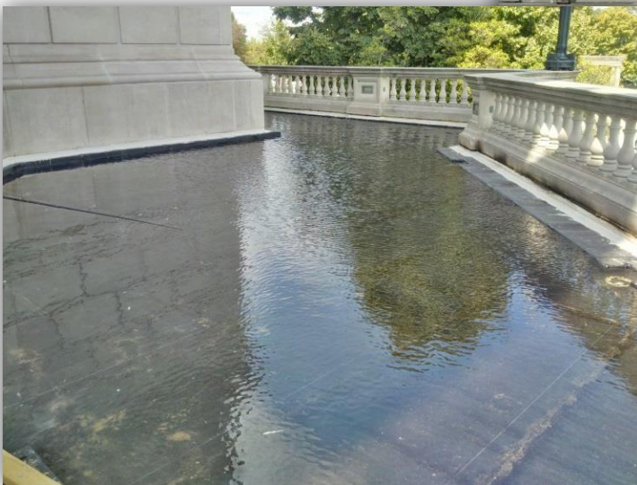
Testing the new waterproofing membrane on the Northeast terrace
